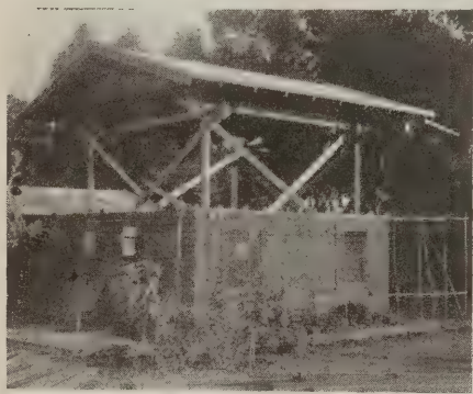
FIG. 1.—ROOF RAISED 8 FT. 7 IN. TO NEW POSITION
